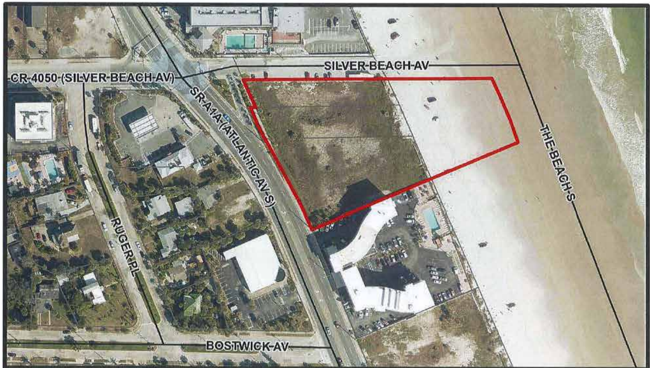
Aerial View of the Property
